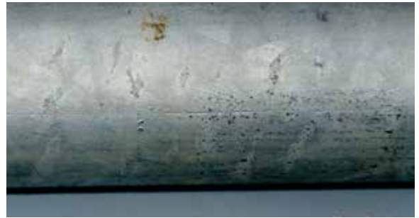
Fig. 3.5.8. Deficient hot-dip galvanizing
