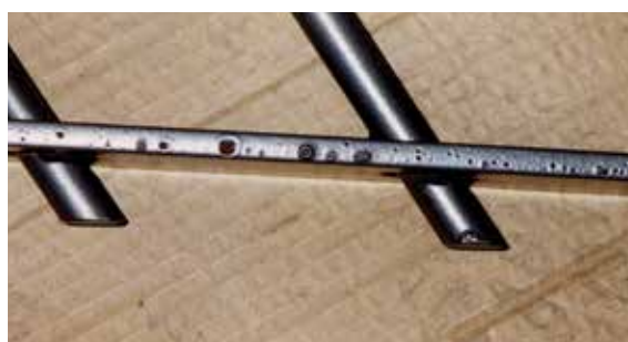
Fig. 3.2.4 Craters in powder coating film due to corrosion
