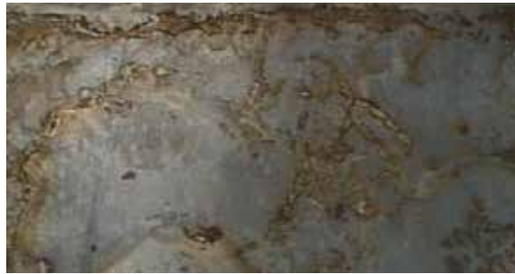
Fig. 1.3.4 Poor rinsing, subsequently stored wet
