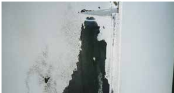
Fig. 2.3.1 Parts of the powder layer slip off
