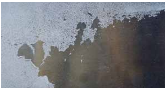
Fig. 3.8.1 Large areas of discontinuity that fail to exhibit a paint film
