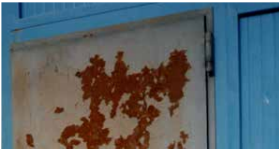
Fig. 5.2.3 Scale, flash rust, white rust
