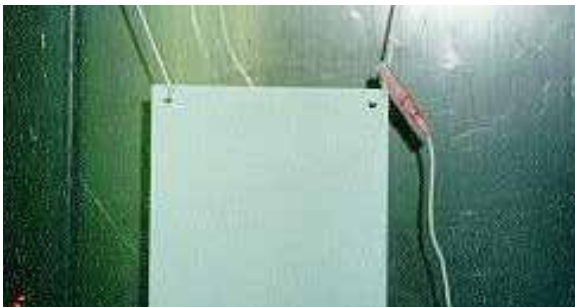
Fig. 2.3.3 No grounding or inefficient grounding
