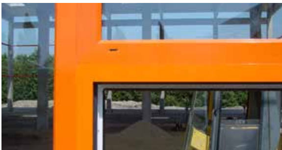
Fig. 4.1.1 Different color due to varying layer thickness
